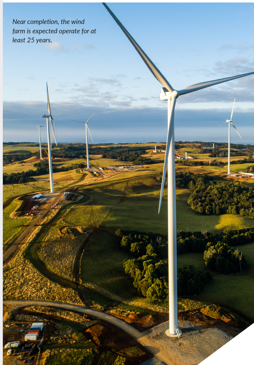
Rehabilitation works are underway onsite to restore the land to pasture for cattle grazing.
